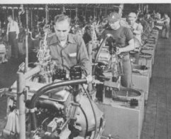
Chevrolet tests an engine while it runs as a unit.
