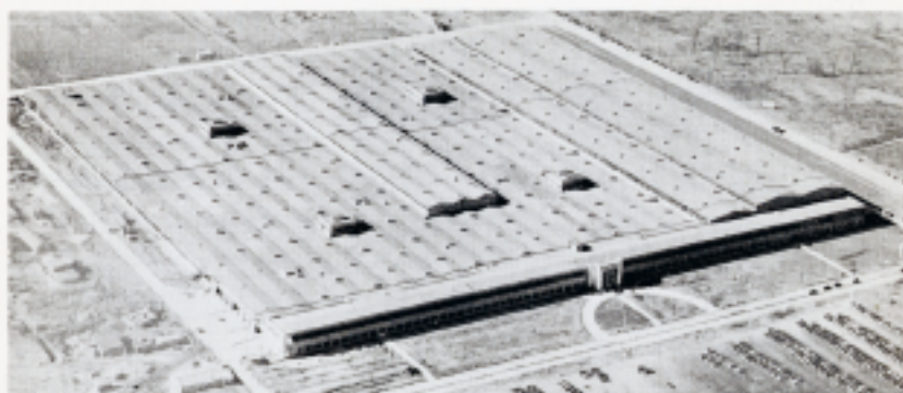
The new automatic transmission and sheet metal parts plant, Cleveland, Ohio
