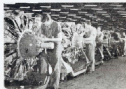
Assembling P & W engines
